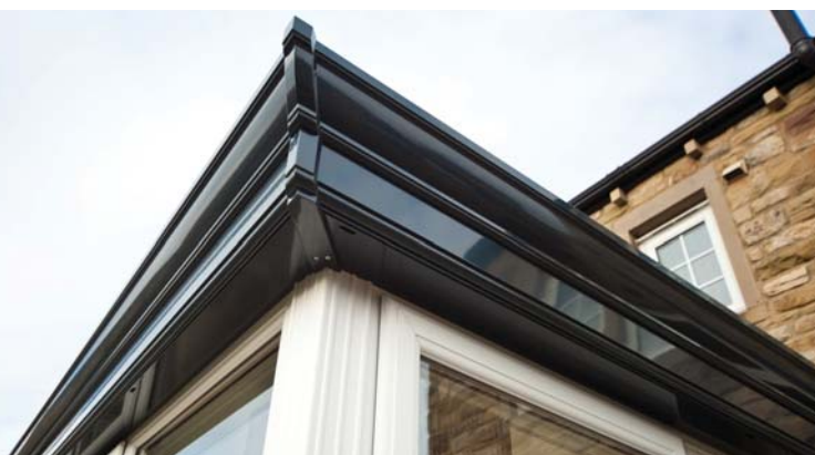
LivingRoof features black pvc gutter as standard - but you can upgrade to this Cornice section to create a subtle difference
